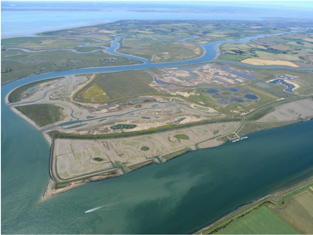
Photo 3 Flood protection and wetland restoration on Wallasea Island, Essex (RSPB)
