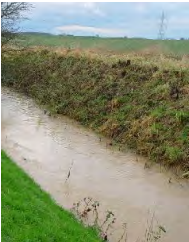
Oldfleet Drain after heavy rain fall.
