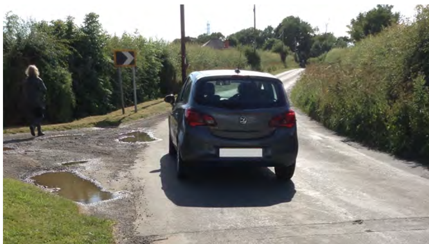
Car on blind bend, with little space to spare with potholes on both sides of the road.
